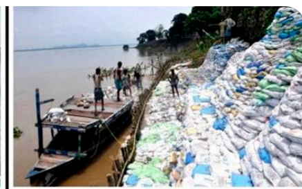
Photo 5 Placement of MacBags™ on the river bank
